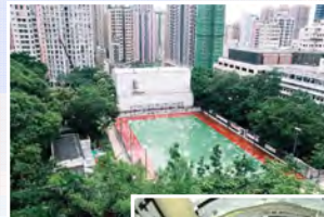
Specially built noise enclosure
