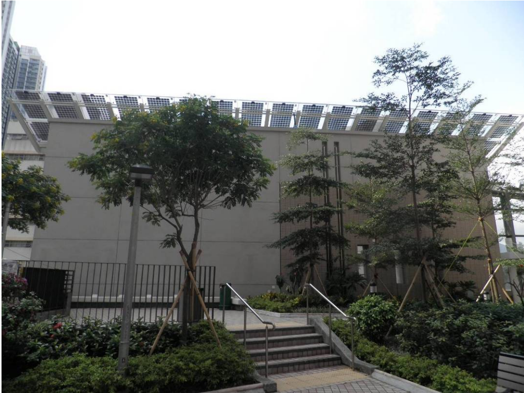
Photo 2: One of the landscaped areas of Yau Lai Estate (with photovoltaic panels installed on the rooftop)
