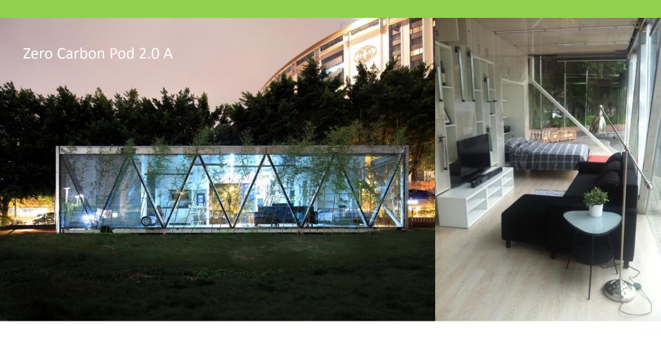
40 square meters 4kw/h Thin film type solar panel 200L phase change solar water heater Ipad control
